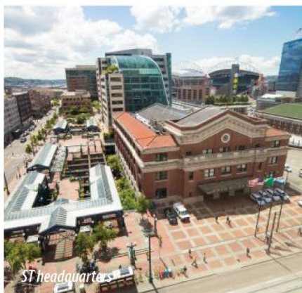
SCC 30 - Support Facilities
